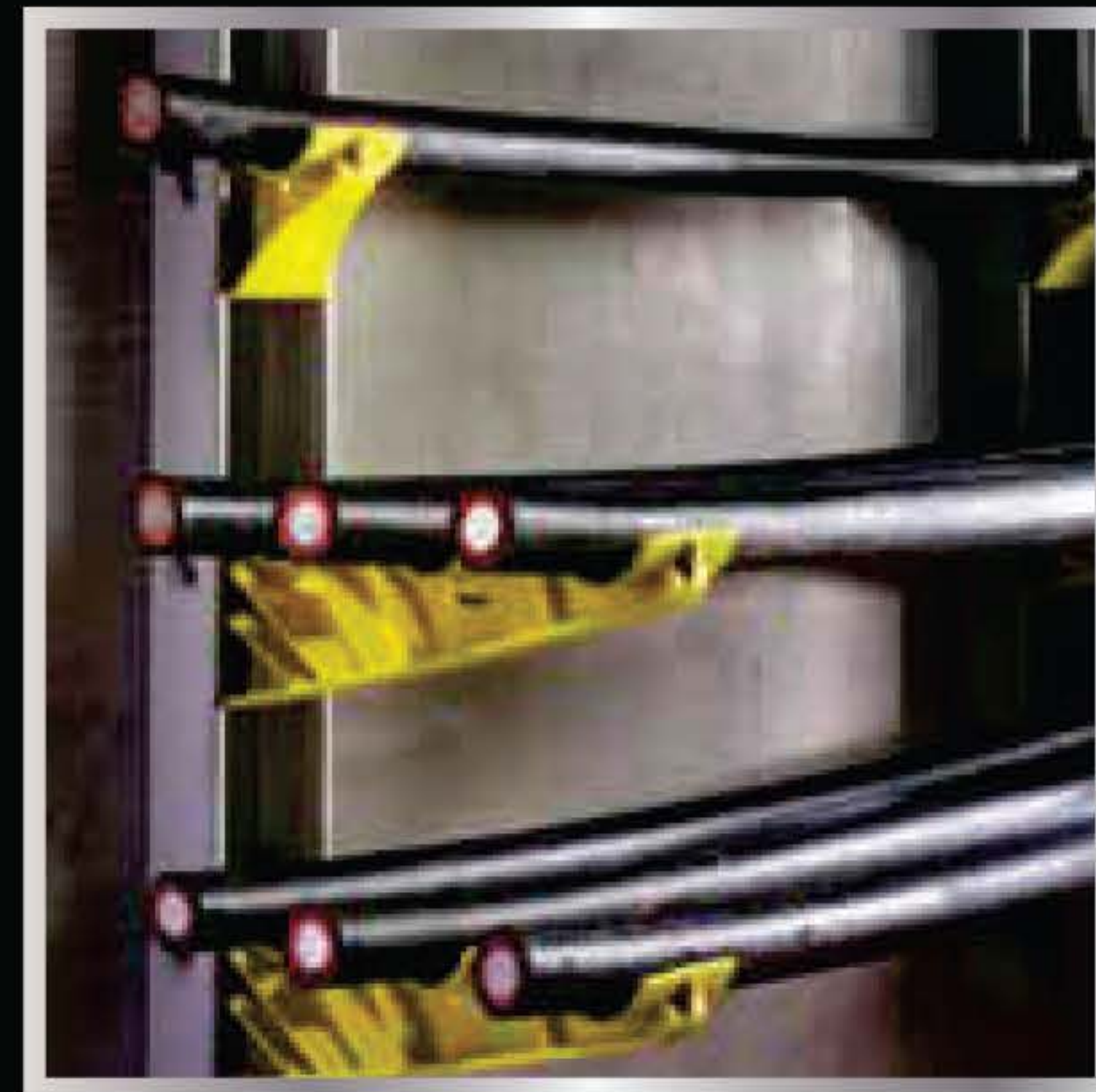
BNT Series Nonmetallic Cable Support Arms Installed in A Nonmetallic Stanchion
